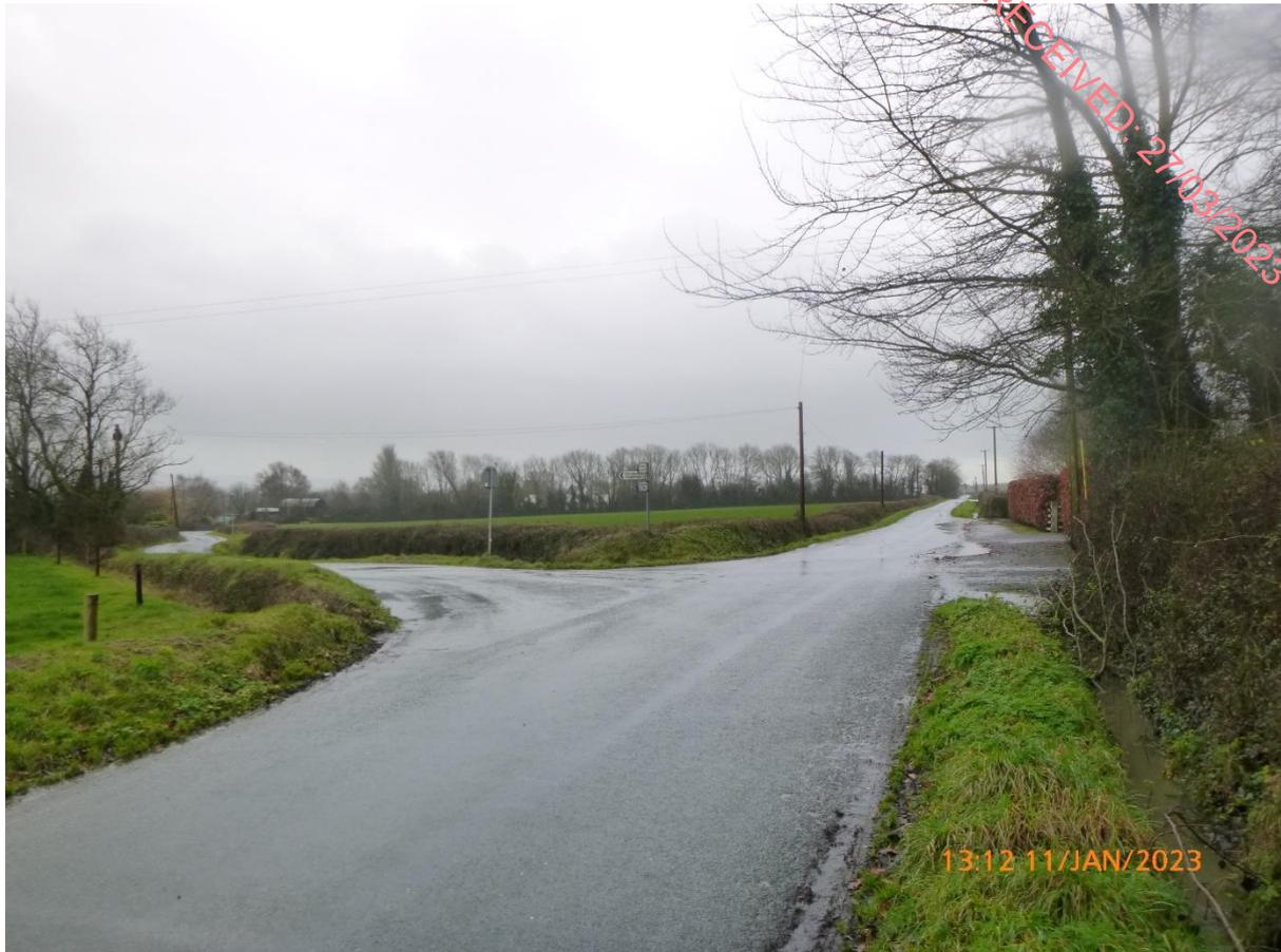
*Figure 12-6: L3036/ L3036 3-arm Stop-controlled Junction (major arm to right, minor arm to left)*
